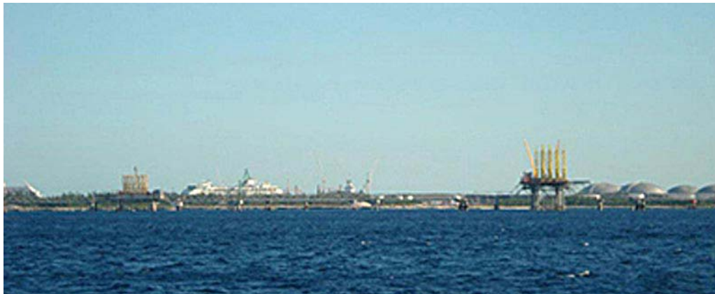
Freeport—BORCO Oil Terminal
