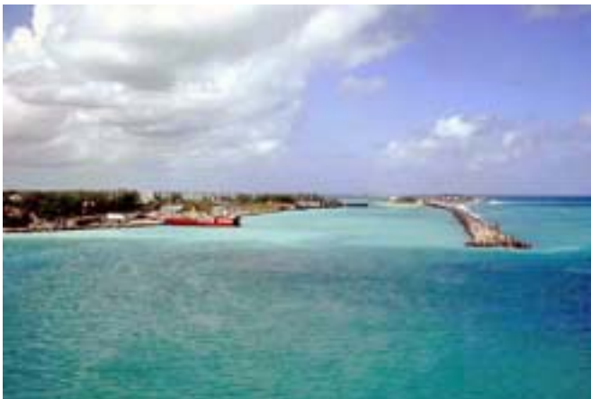
Arawak Cay—West Breakwater
