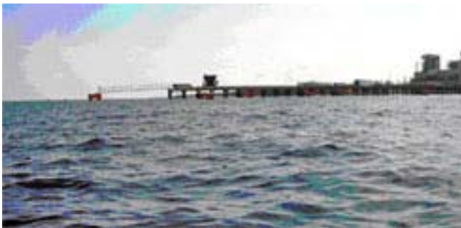
ITABO Fuel Pier
