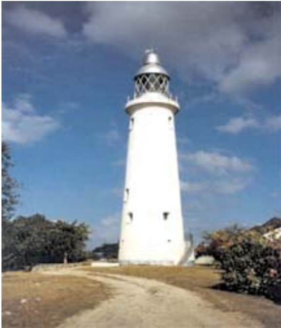
South Negril Point Light
