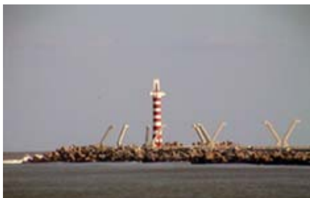
Coatzacoalcos Entrance Light on the breakwater
