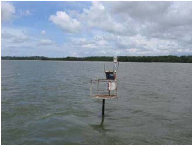
Light marking a Submerged Obstruction near Puerto Santo Tomas de Castilla (E of Main Channel)
