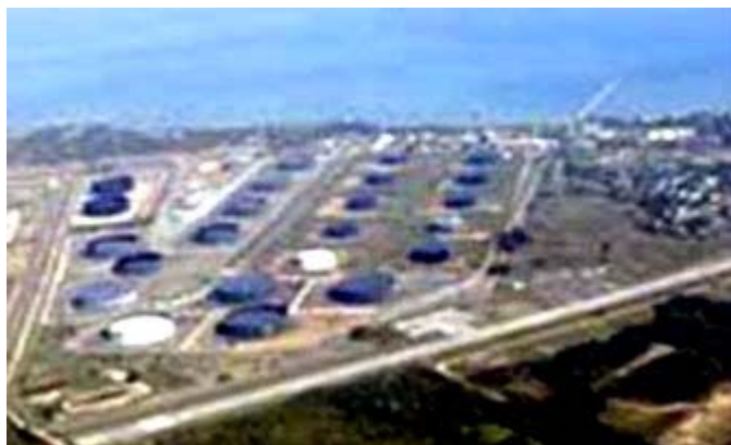
Covenas Tank Farm
