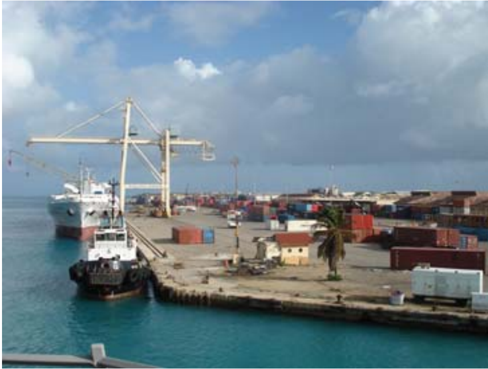
Parden Baai—Container Terminal
