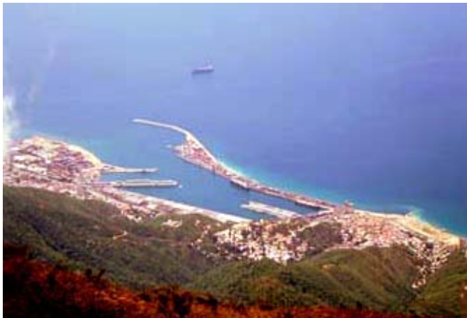
Puerto La Guaira (aerial view)
