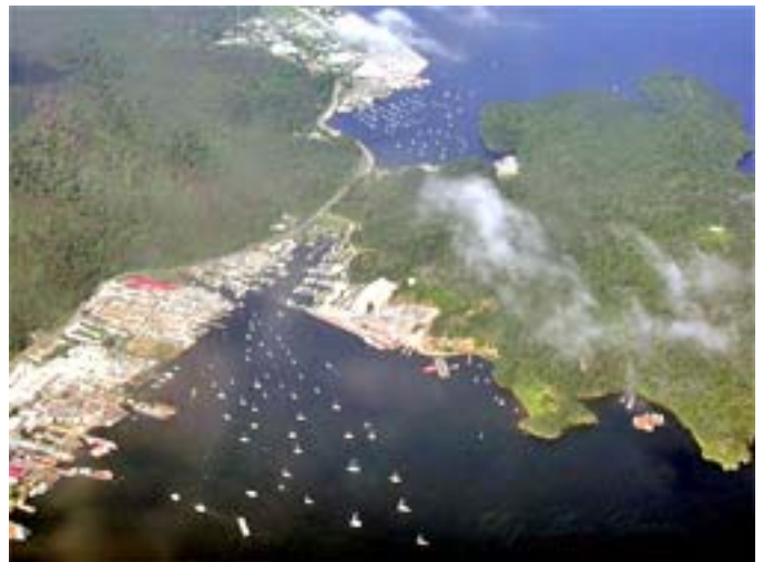
Chaguaramas Terminal Wharf (center)
