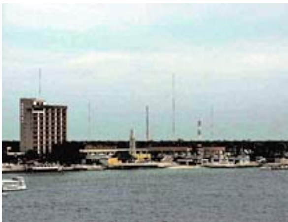
Cozumel—Conspicuous Hotel and Water Tower
