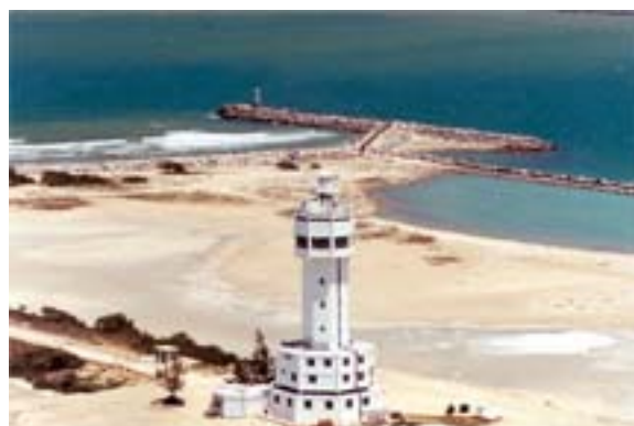
Altamira Light (foreground) and breakwater
