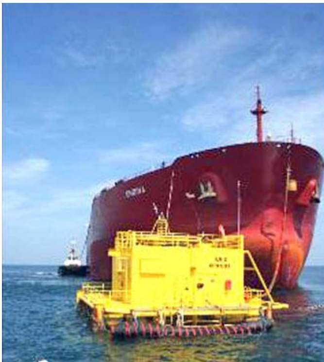
Covenas Tanker Loading Unit (TLU-2)
