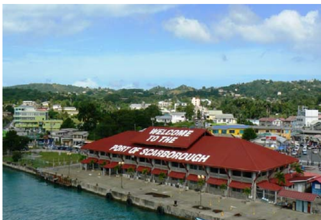
Scarborough Port Terminal
