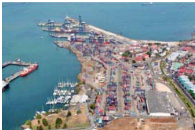
Puerto Cristobal—Piers 6 through 10 (upper) and Pier 16 (left)
